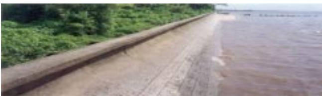
Figure 6 - “Sea Walls,” used to keep the sea water out and provides a difference of head for drainage purposes during low tide.
