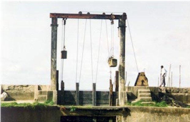
Figure 12 - Sluice Gate used for drainage by Gravity, locally called a “Koker.”
